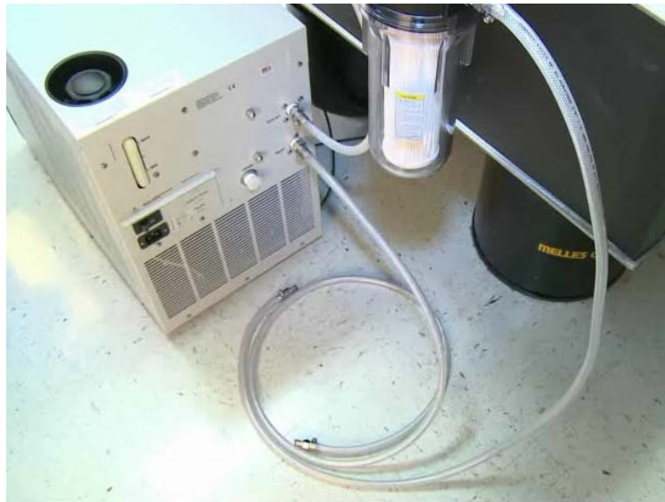
Figure 4-4. Chiller Assembled with Water Hoses and Filter
